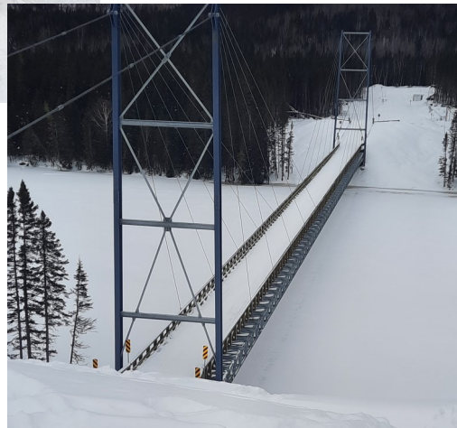
Day 4, Picture of the bridge at the 49th Parallel.
